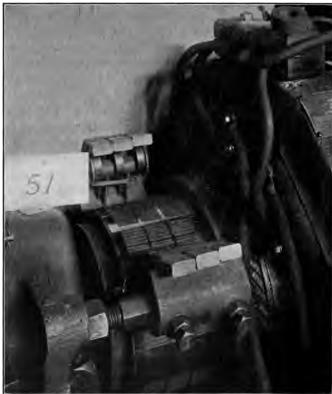
FIG. 98.—Commutator having a burned surface as a result of severe short circuits while not in operation. Note also the condition of the surface preceding the formation of ridges due to lack of brush stagger.
